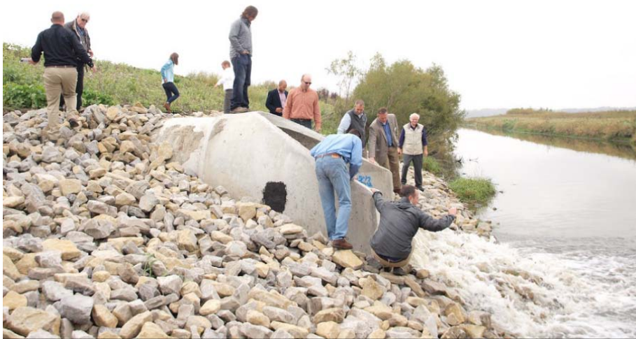
Ducks Unlimited supporters and volunteers open the flood gates to restore water to the wetland area which had been drained. Photo courtesy of DU.
