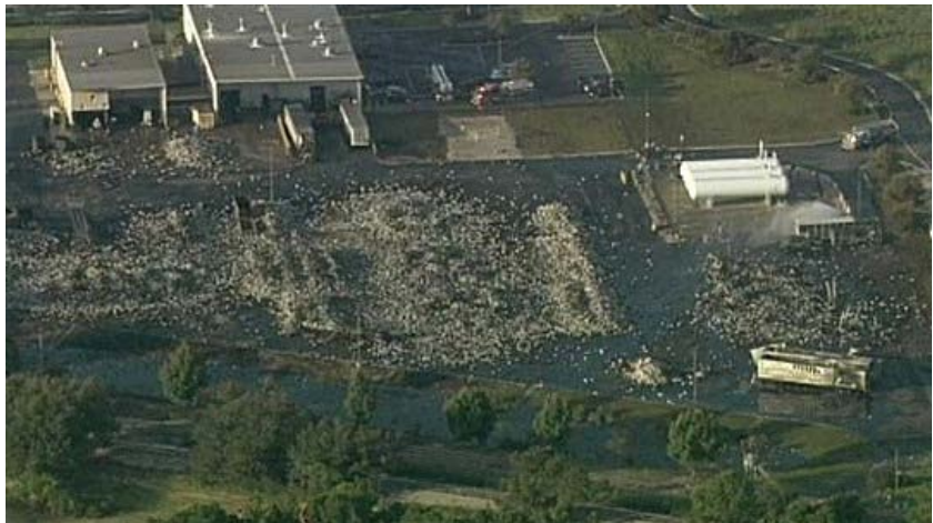
An aerial view of the Tavares propane plant showing thousands of propane tanks littering the ground after the explosion. These photos were taken by Michael Ellis, and this view was being shown on the local TV station when he snapped a photo of the TV screen!
